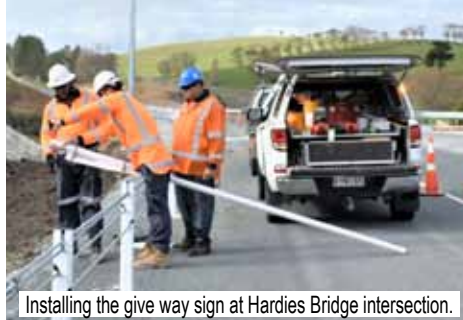
Installing the give way sign at Hardies Bridge intersection.
